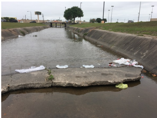
Figure 1. Stewardship Site: Spring Creek Storm Drain, Victoria, Texas
